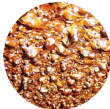
Varnish on reservoir ceiling (Stalactites)
